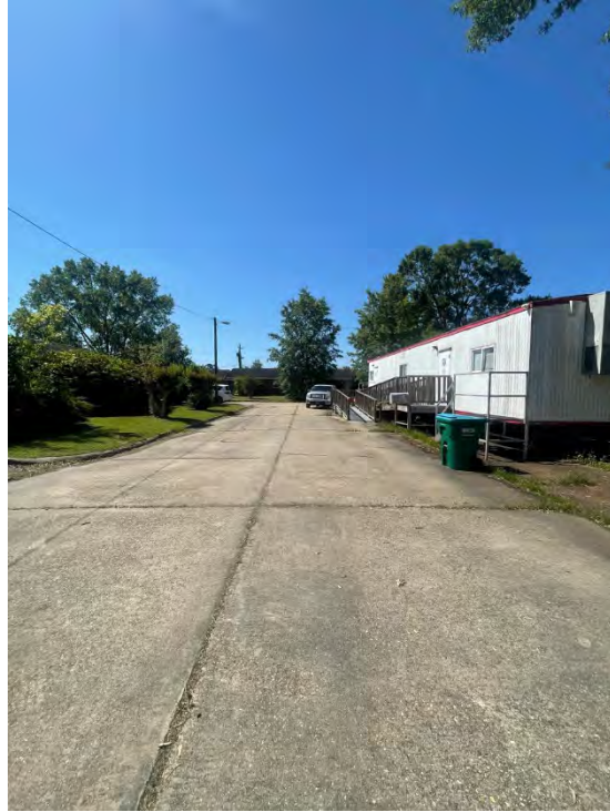
Photo 1. View of existing DSHA administrative building at located at original facility at 600 Eugene Street.
