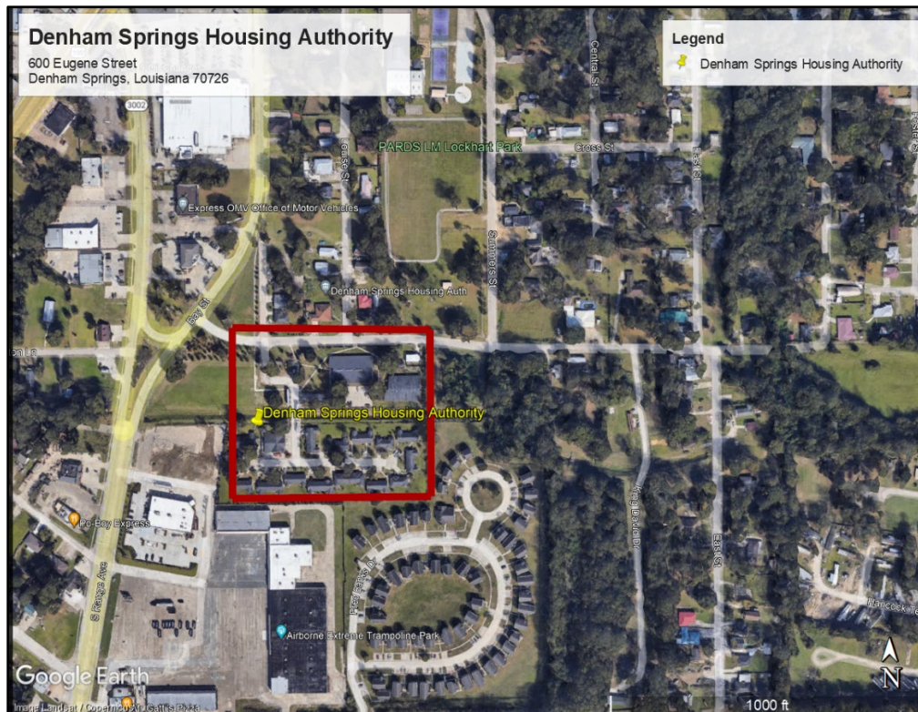
Figure 7 – Aerial view of the damaged Denham Springs Housing Authority.
